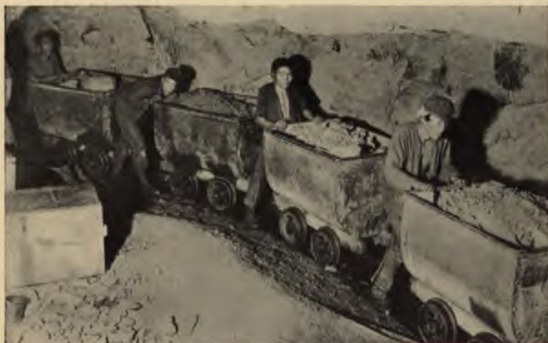
TRUCKING THE ORE TO THE SHAFT
